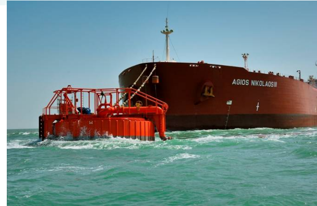
Single Point Mooring
